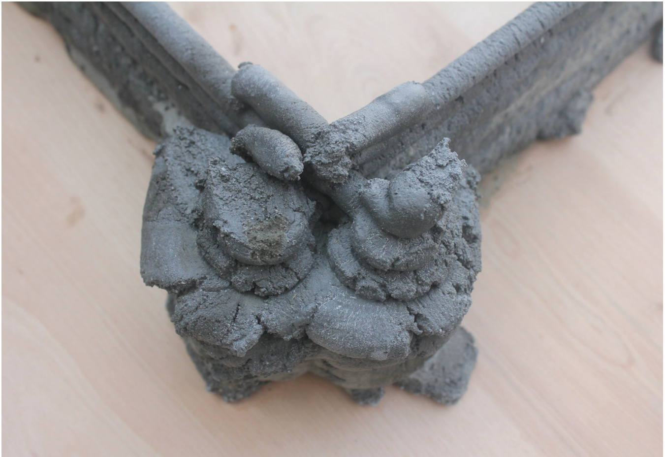
Figure 2. 3D printed concrete lines are extended past one another in order to create an ornament at the corner.
